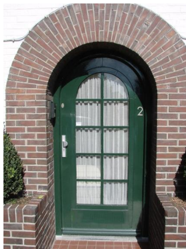
this is not a door
